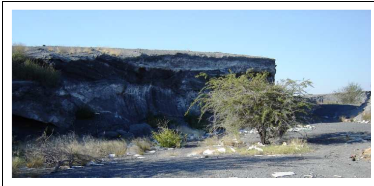
Plate 3.4: Contractors at Berg Aukas have been removing slag and fly ash for brick making from the dump leaving a dangerous, unsafe working face. It has also been found that this ash and slag are toxic.
