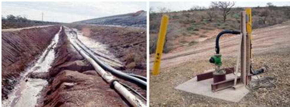
Figure 17: Seepage collection ditch (left) and a seepage well (right)
