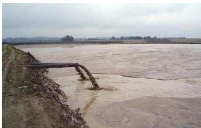
Figure 9: Single point discharge at Glebe Mines, Derbyshire, England
