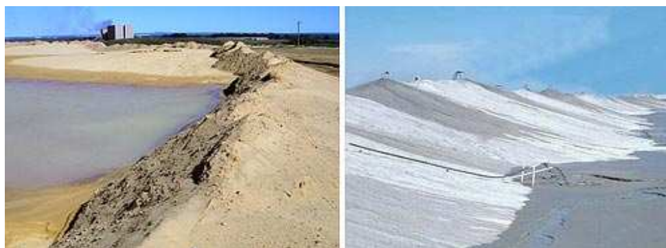
Figure 15: Loss of freeboard (left) and high freeboard (right). (Right picture courtesy of Anglo America)
