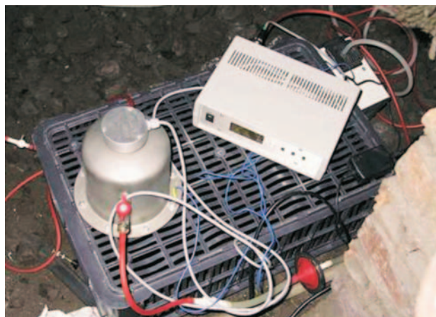
Fig. 4-6. Measuring system RM-3 – continual measurement of soil gas radon concentration.
