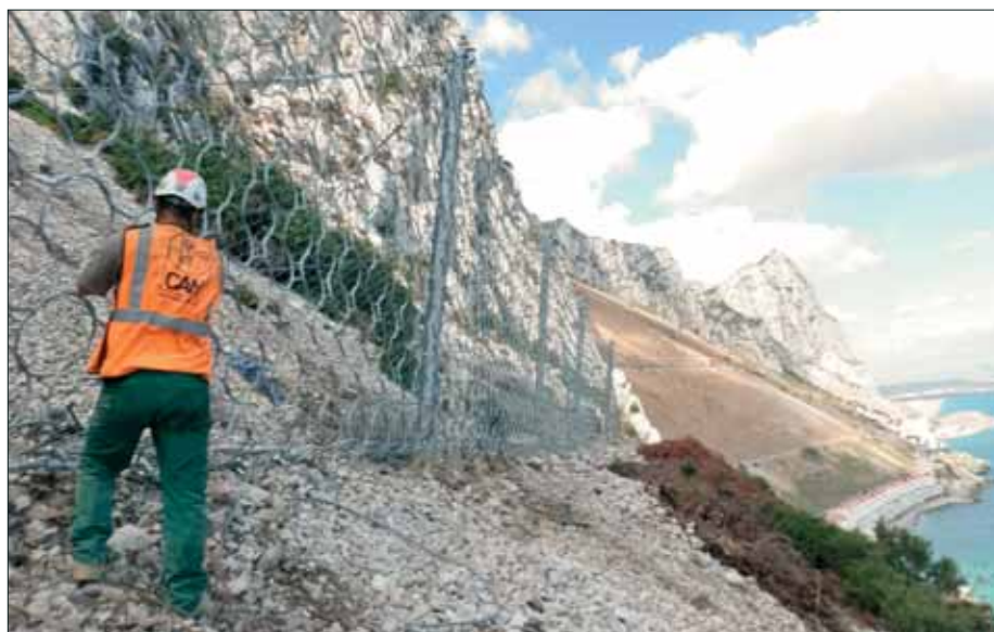
Fig. 5.61 Dynamic barrier – ring panel. Source: Maccaferri
