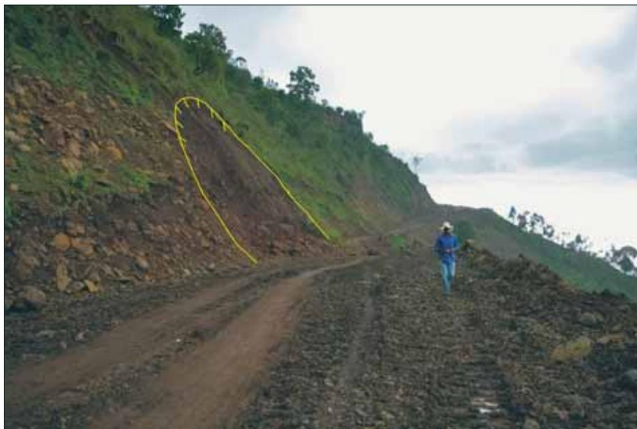
Fig. 5.38 Boulders and debris fall to debris slide in the Gambelo – Mejo road cut
