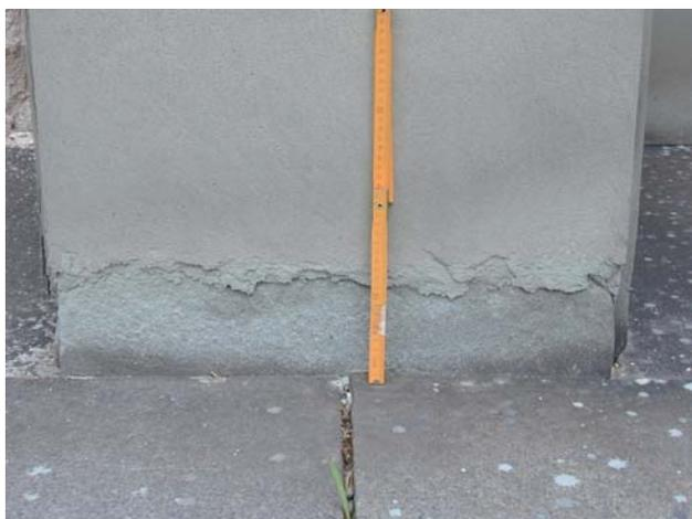
Figure 16. Exfoliation of the Godula Sandstone caused by a combination of moisture and frost. Basement of the Military Academy in Brno (20<sup>th</sup> century). Photo P. Pospíšil.
