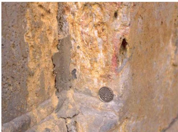
Figure 15. Gradual weathering of the Maletín Sandstone caused by moisture and frost action in the basement of a seventeenth-century structure in the town of Olomouc. Photo by P. Pospíšil.
